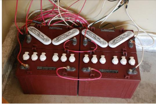
*Batteries C and D at top, E and F lower. C and D are in series to make 24 V, as are E and F. These two chains are wired in parallel to each other. Looking somewhat different (E/F are T-1275+), the internal construction of all four batteries is identical.*
