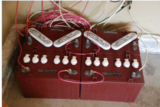
*Four golf-cart batteries used in my off-grid home PV system. Each is 12 V, 150 A-h, thus 1.8 kWh of storage.*
