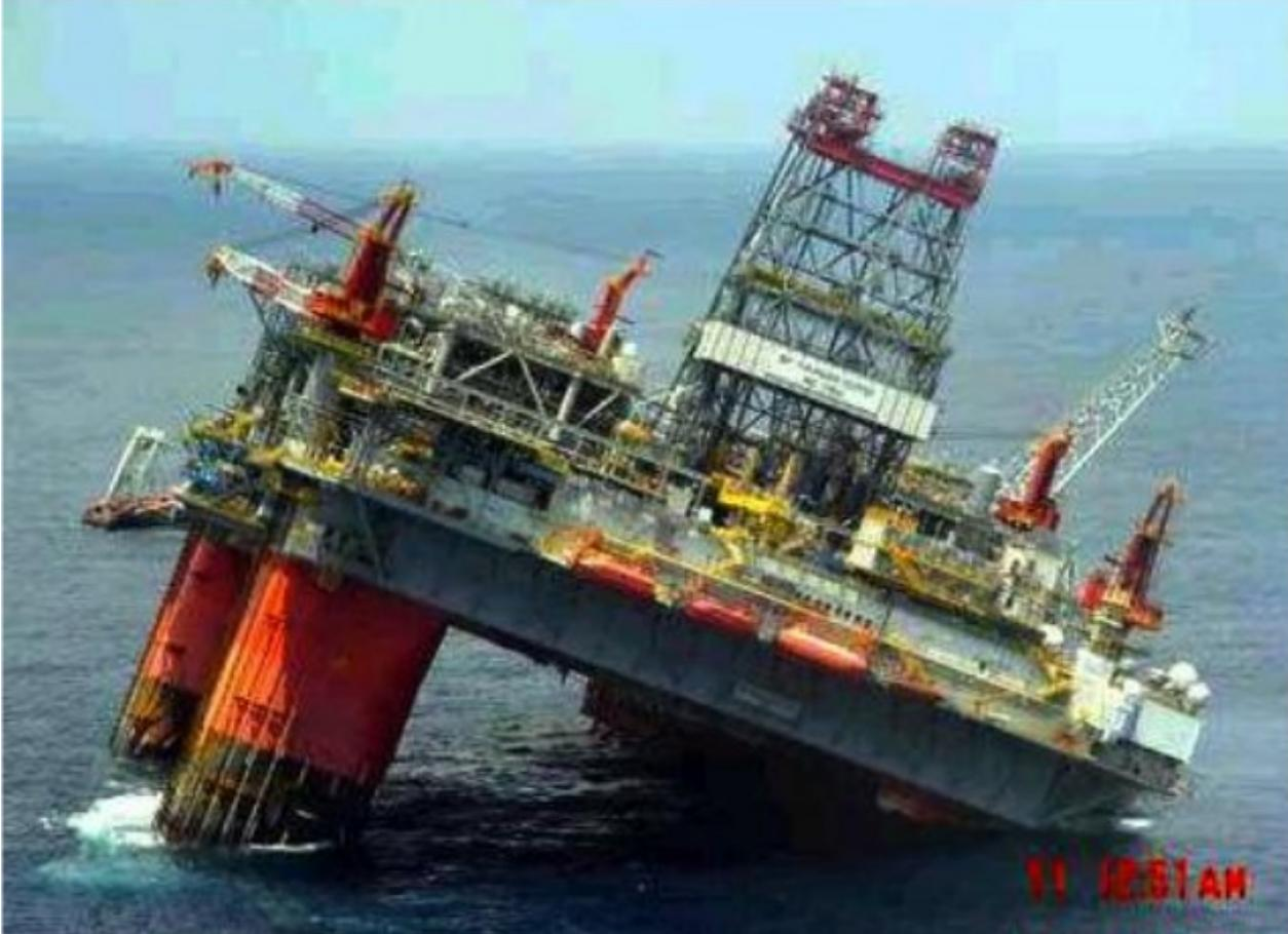
Due to a faulty ballast valve, water entered the ballasts and expensive work had to be carried out to remedy all the damaged parts.
